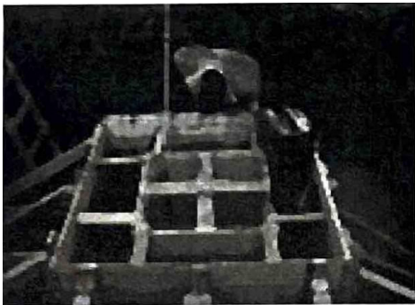
Fig.63 Montare cofraj
